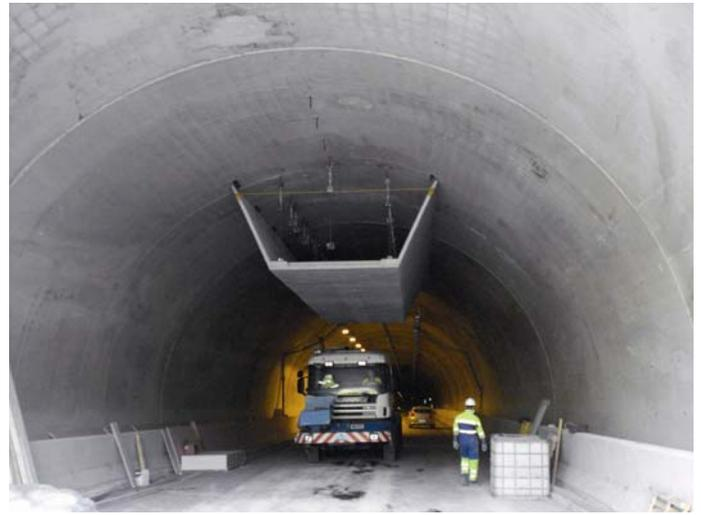
Figure 2 The Suspended Emergency Exit
