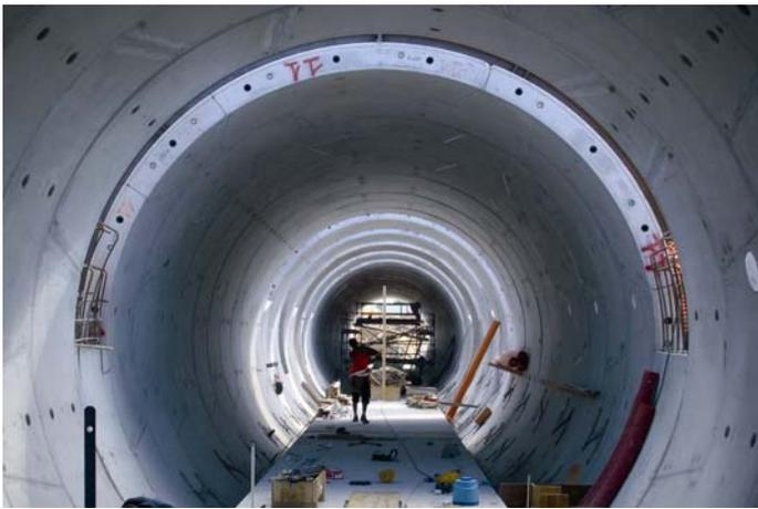
Figure 12 The construction of the test tunnel at the Montelibretti school for fire-fighters
