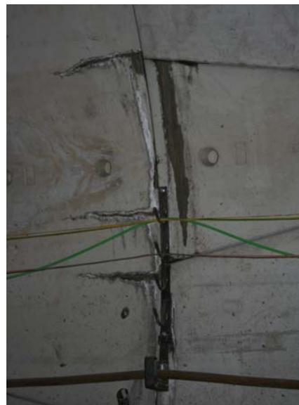
Figure 2 Longitudinal cracks in the prefabricated segments of TBM driven tunnels
