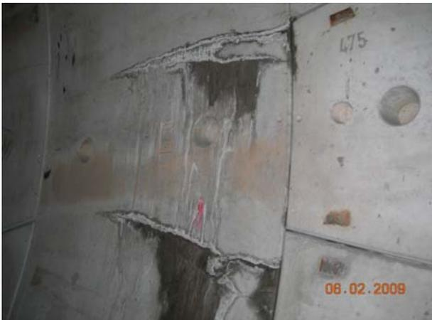
Figure 3 Cracks in the prefabricated concrete segments of TBM driven tunnel
